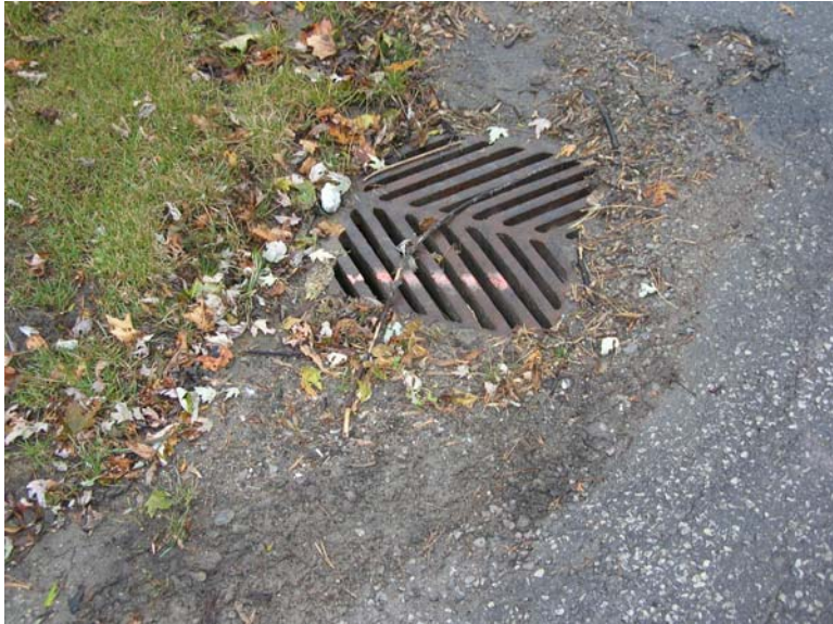
Photograph 1: Typical Catch Basin Inlet Lake Drive North
