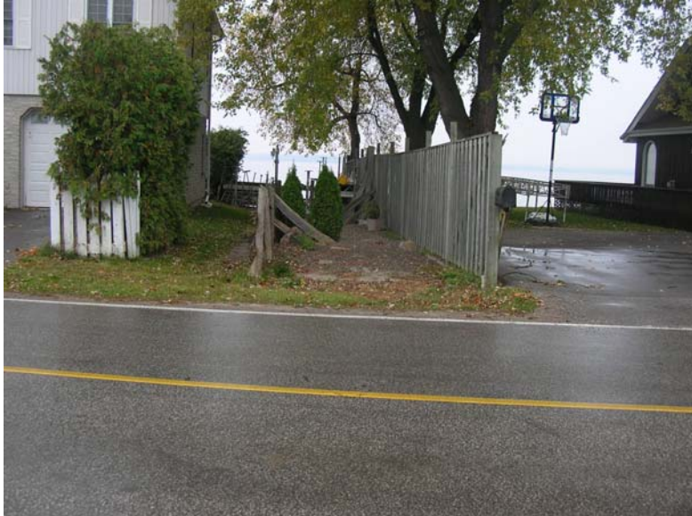
Photograph 2: Typical Outfall Location Lake North Drive
