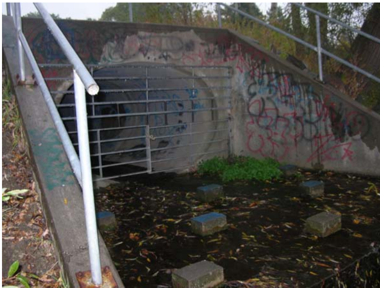
Photograph 4: Major Storm Outfall
