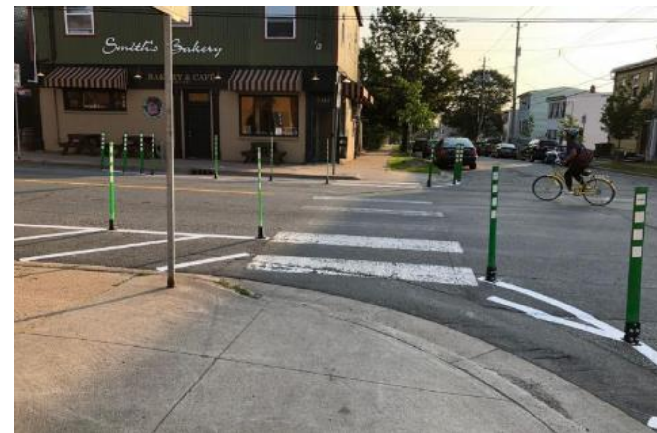
Temporary Curb Extensions
