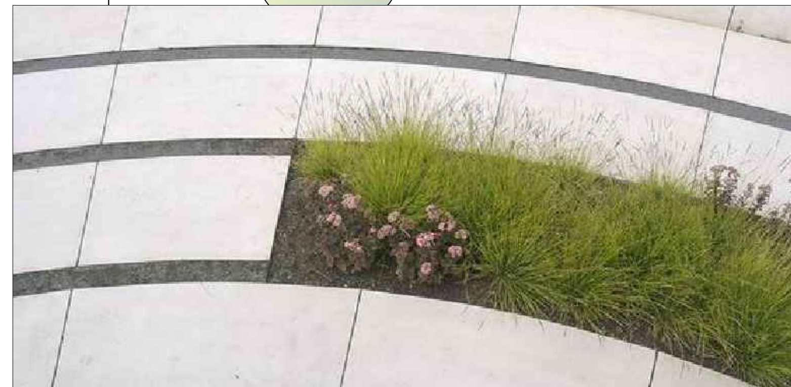
Coloured Concrete Paving Bands
