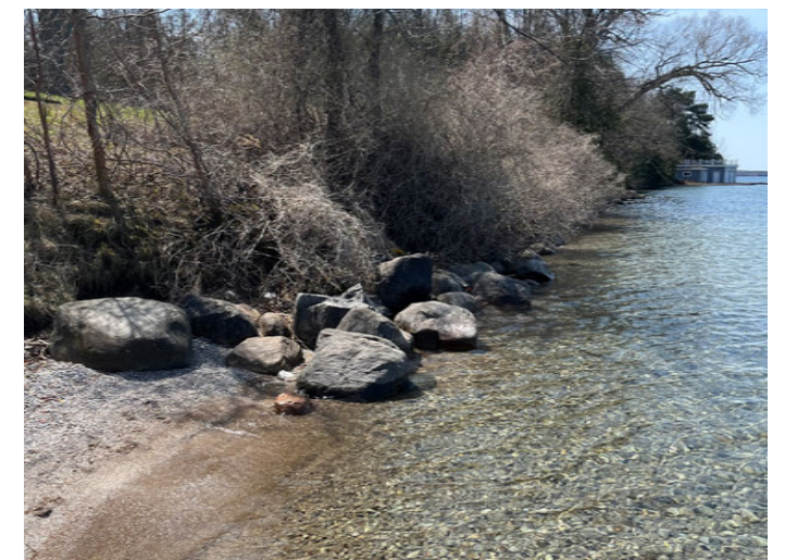
Existing shoreline conditions along North Gwillimbury Park
