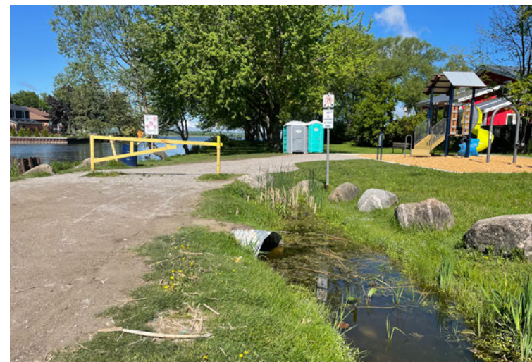
Playground and drainage culvert
