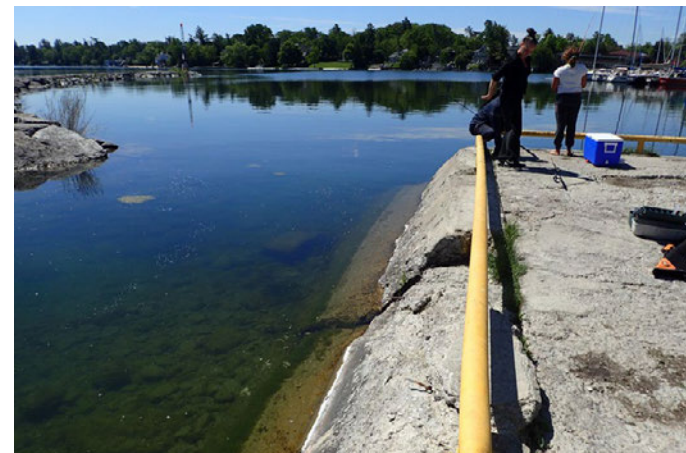
Existing shoreline conditions along Malone Wharf
