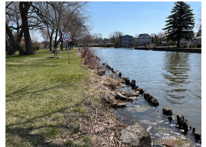
Existing shoreline conditions along Young's Harbour Park
