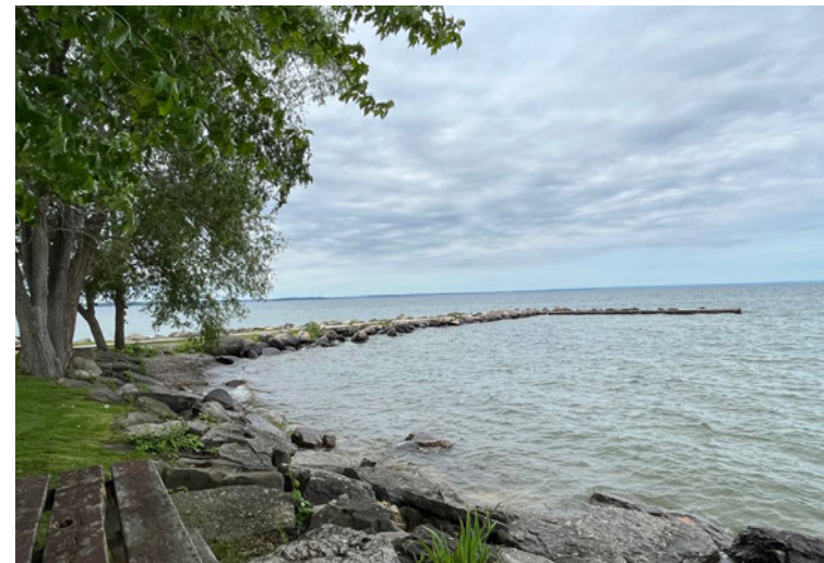
The wharf at Willow Wharf Park
