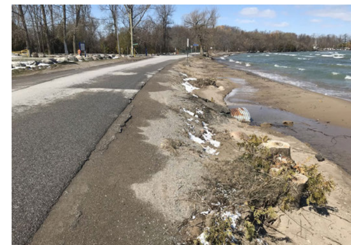
Existing shoreline conditions along Franklin Beach
