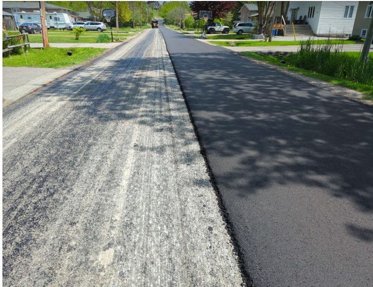
Two-coat microsurfacing:
