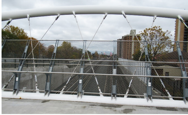
Figure 2 – Localized fencing around structural members
