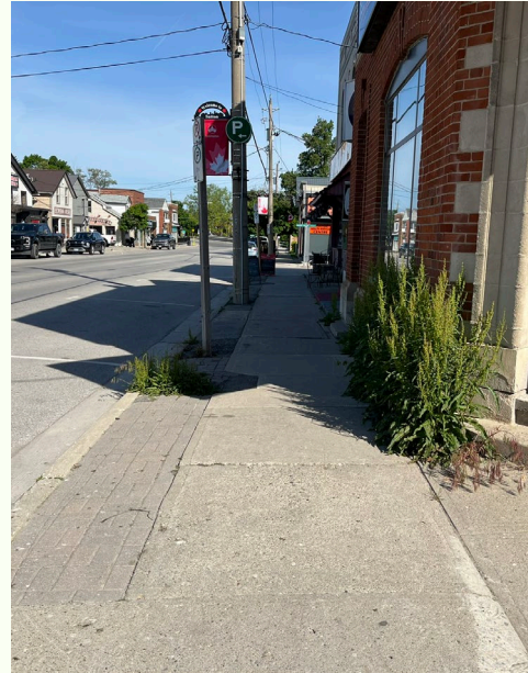
SUTTON, ON HIGH ST. PRE-CONSTRUCTION
